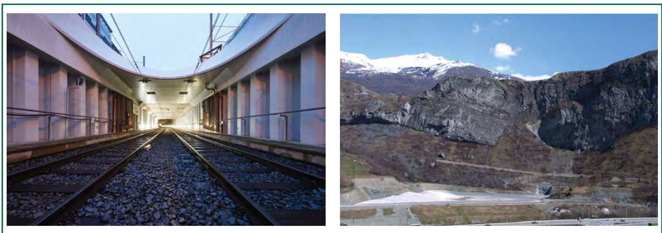
Figure 1-1 Comparison of modelling requirements – building on the left (photo: Implenia/Bernd Schumacher), ground on the right (photo: Implenia)
